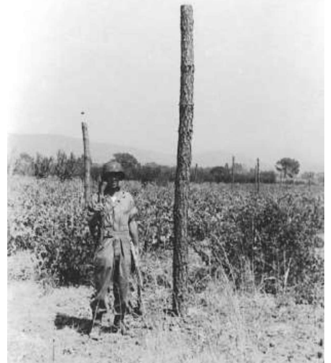
Zane Graves stands by Rommel's asparagus, in LZ-O, intended to destroy the gliders as they landed. Under the Service Travail Obligatoire (STO) were young and old French citizens who could not work in Germany as forced laborers were made to put up the poles. When the Germans were not looking they set the poles only two feet into the ground. Gary H. Graves collection
