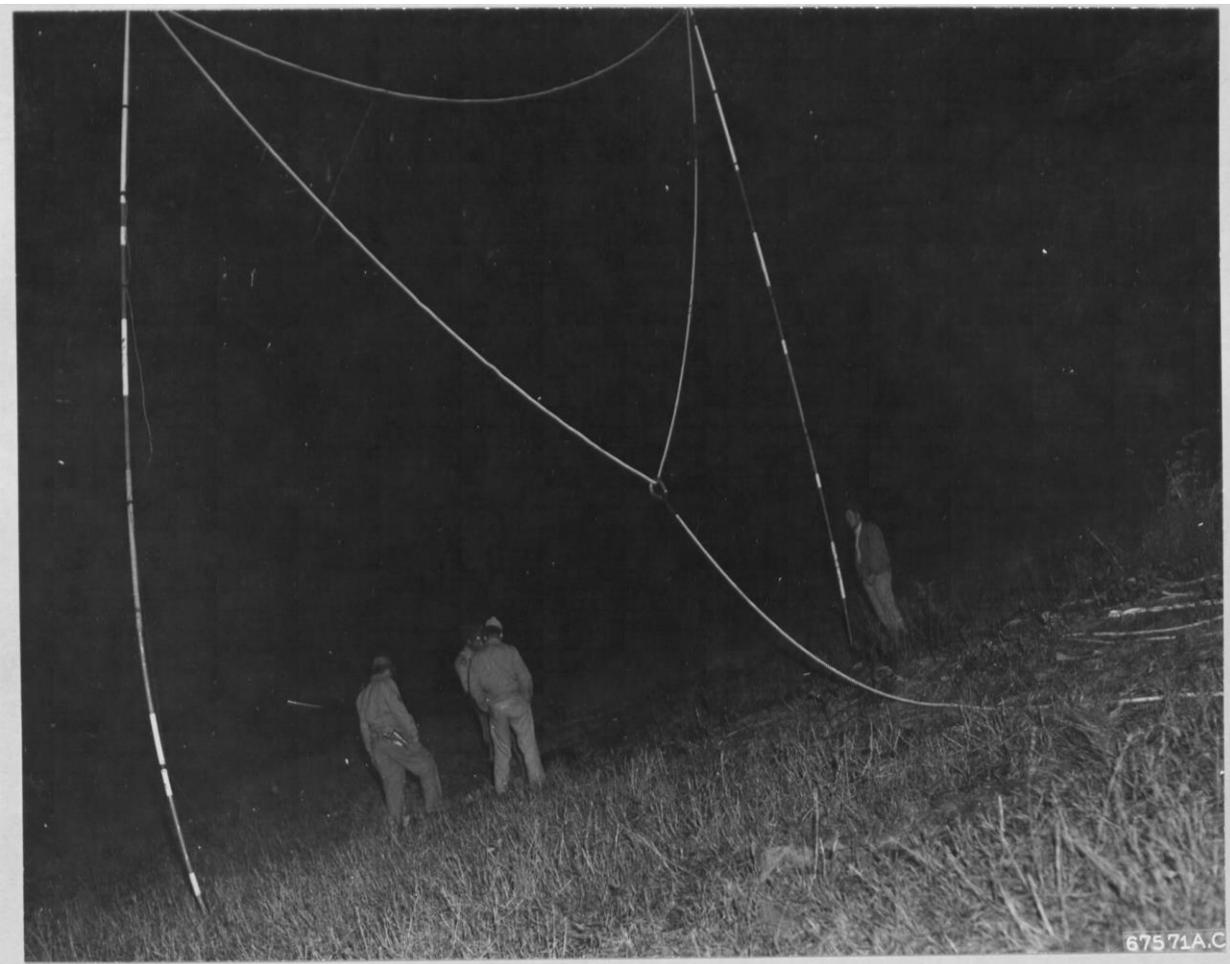
1AC night photo, 24' tall pickup poles w/standard pickup line loop. Four men would be four of those previously listed.
